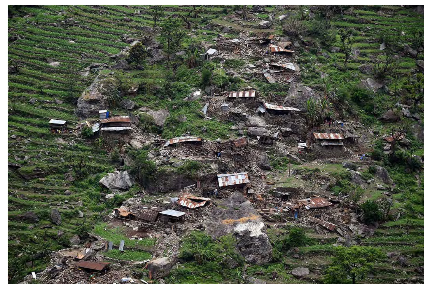
Earthquake-damaged houses in Gorkha District are seen from an Indian Army helicopter - ( Sajad Hussain/AFP ) www.ibtimes.co.uk
