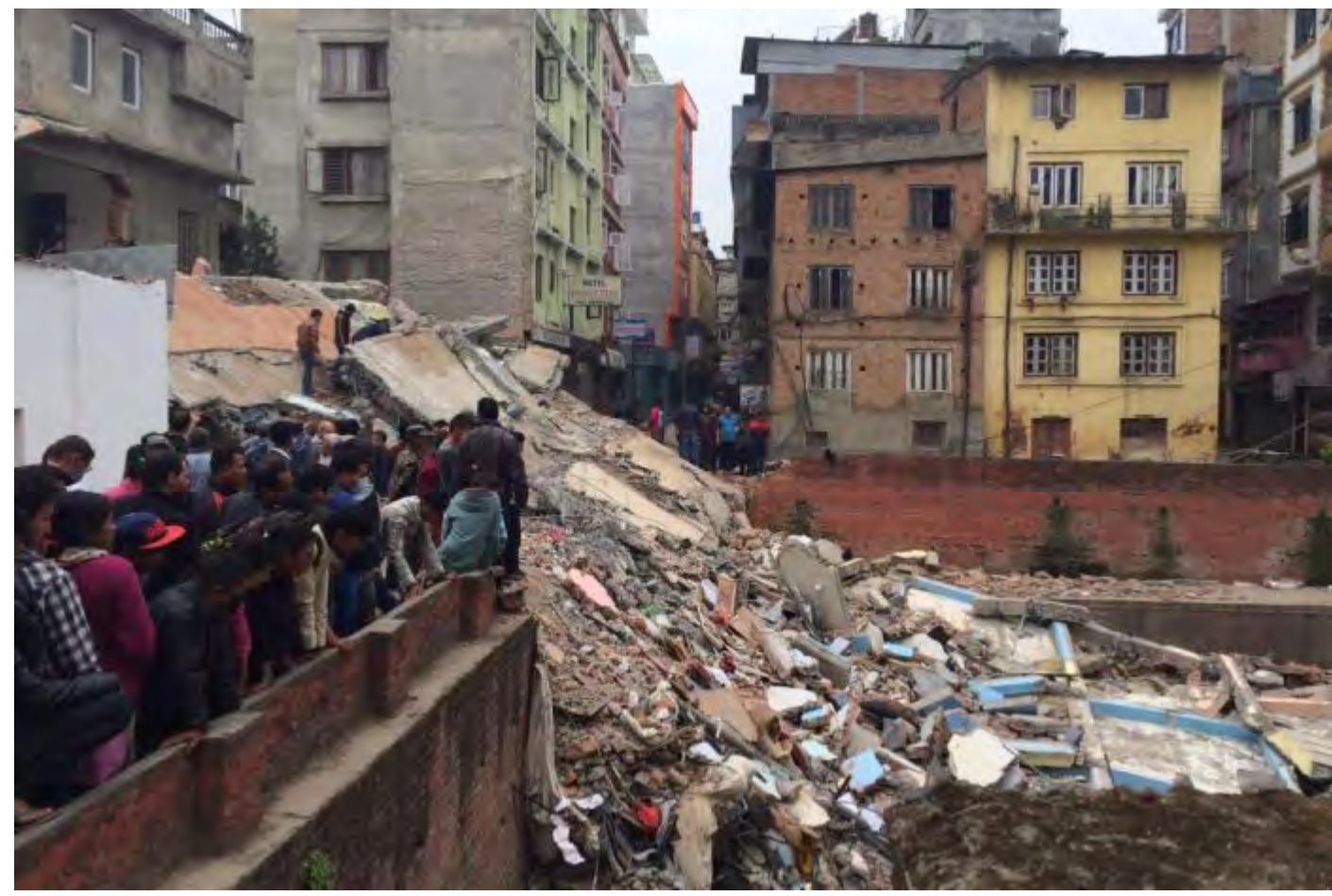
Collapsed building in Thamel, Kathmandu. - www.abc.net.au
