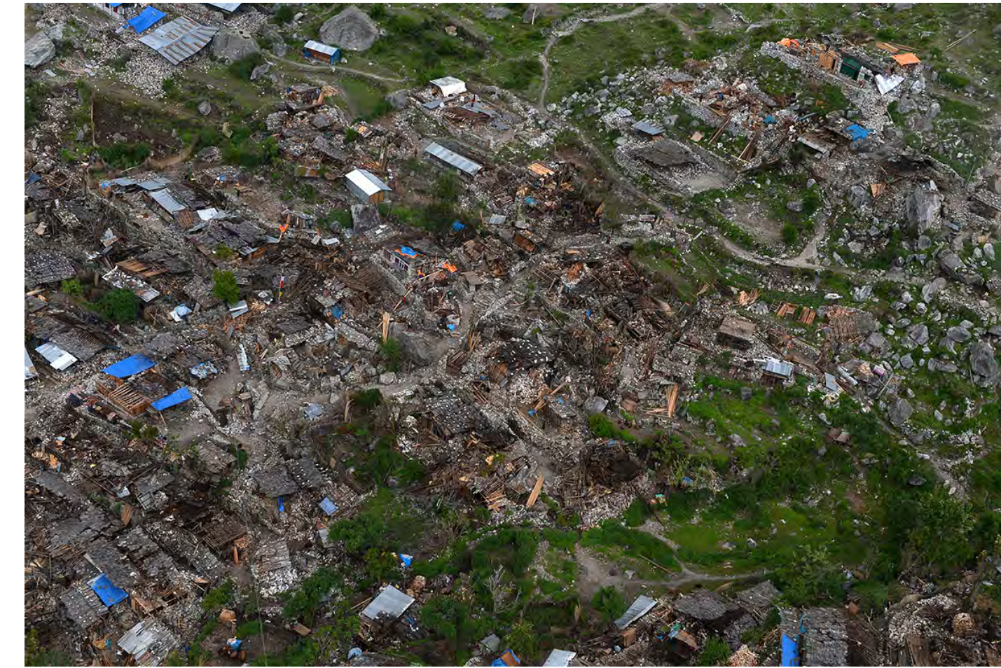
An aerial photo of earthquake-damaged houses at Kerauja village, in northern-central Gorkha District - ( Sajad Hussain/AFP ) www.ibtimes.co.uk
