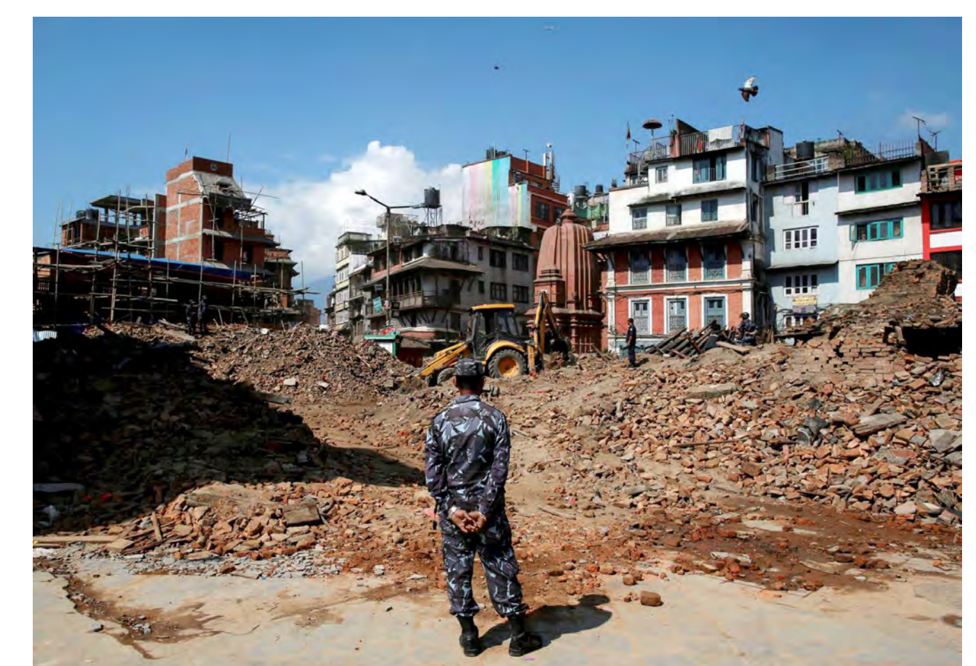
The Nepalese police looks on as an excavator is used to dig through rubble to search for bodies, in the aftermath of Saturday's earthquake in Kathmandu. - time.com
