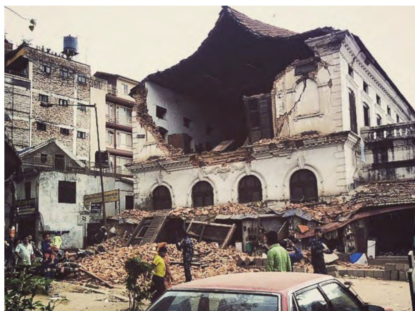
PHOTO: Damage in the city of Kathmandu after a massive earthquake strikes Nepal. - Instagram_NepalQuake , abcnews.go.com
