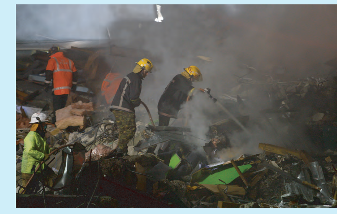
Emergency services team members search for survivors in the rubble of the collapsed CTV building in Christchurch's business district on Tuesday, Feb. 22, 2011. (AP Photo/New Zealand Herald, Brett Phibbs)
