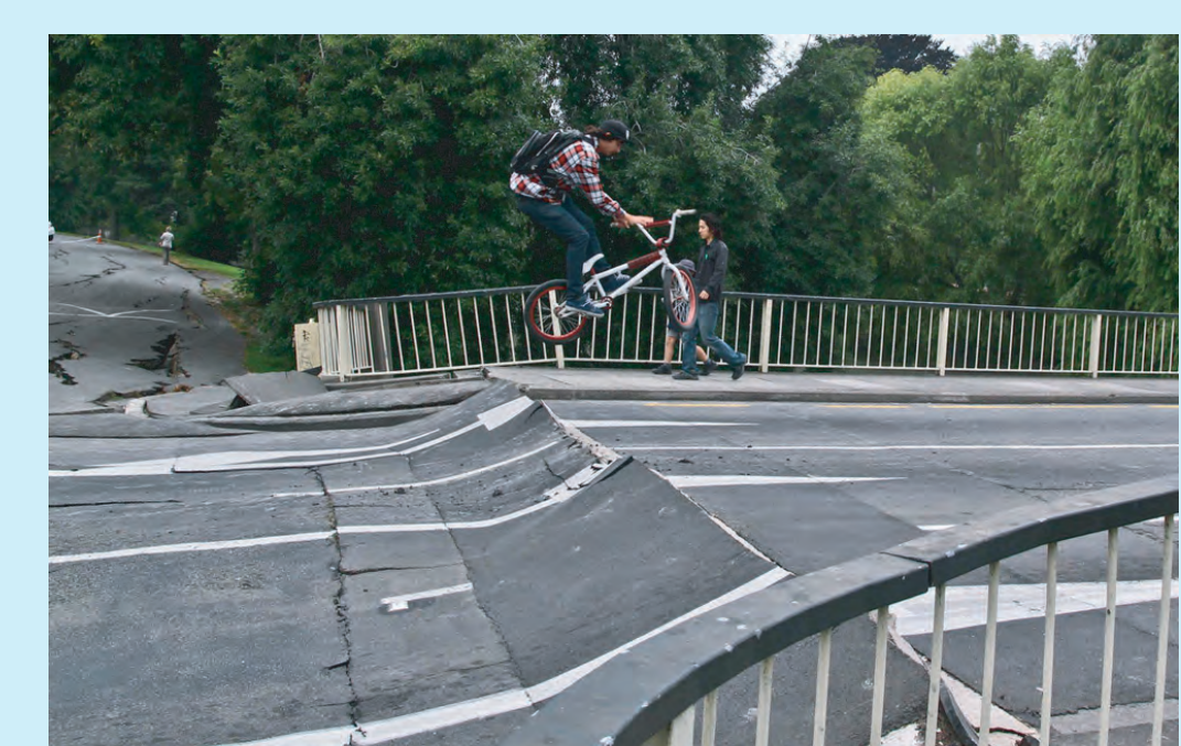
A young man jumps his bike on part of an earthquake-damaged bridge in Christchurch, New Zealand on February 22nd, 2011. (© Asher Trafford)
