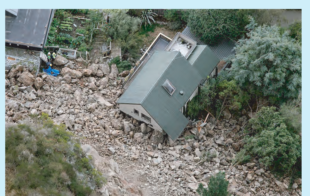
A large landslide lands on a house in Sumner on February 23, 2011 in Christchurch, New Zealand. (Martin Hunter/Getty Images)
