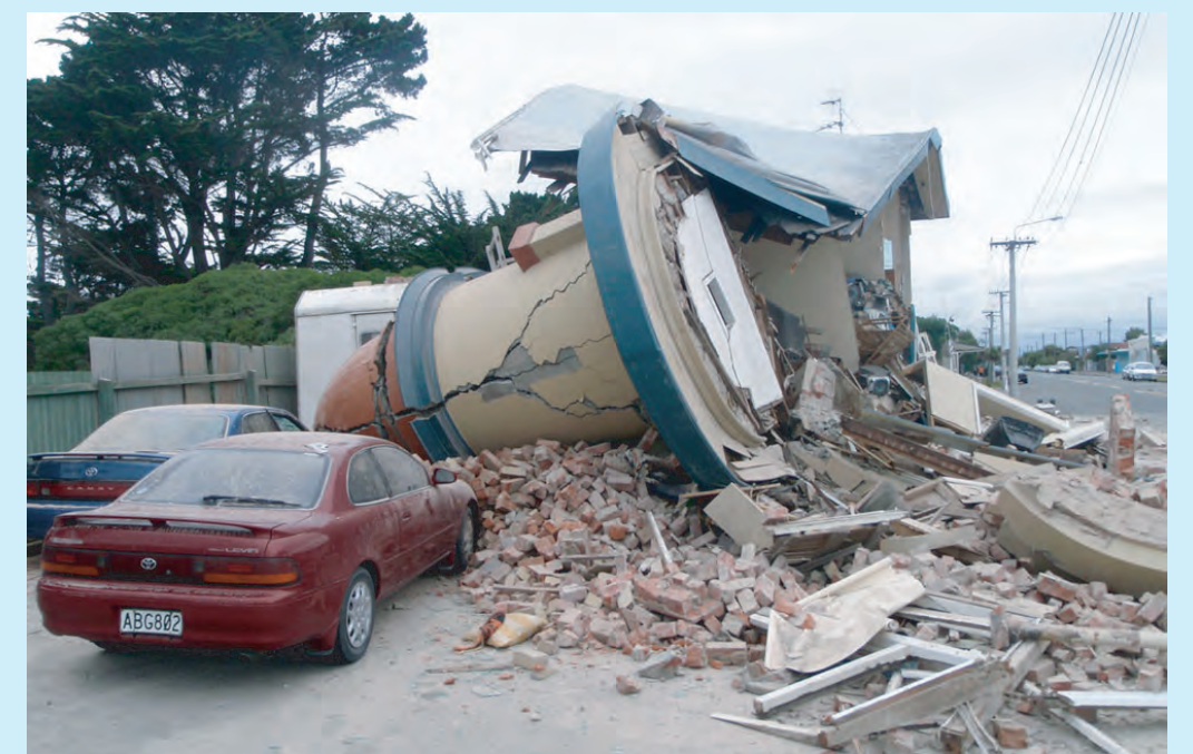
A general view shows a damaged building after an earthquake in Christchurch February 22, 2011. (REUTERS/Jason Tweedie)
