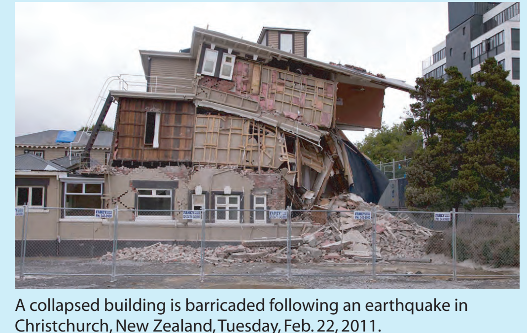
A collapsed building is barricaded following an earthquake in Christchurch, New Zealand, Tuesday, Feb. 22, 2011. (AP Photo/New Zealand Herald)
