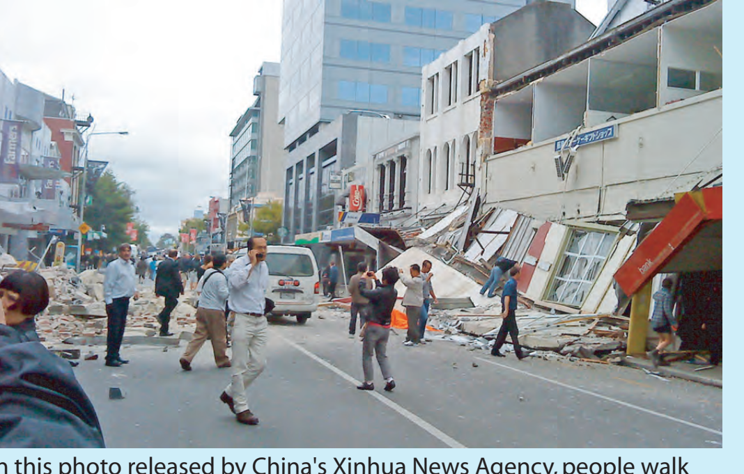
In this photo released by China's Xinhua News Agency, people walk through a street partly covered with rubble after an earthquake hit Christchurch, New Zealand, Tuesday, Feb. 22, 2011. (AP Photo/Xinhua, Pu Rui)
