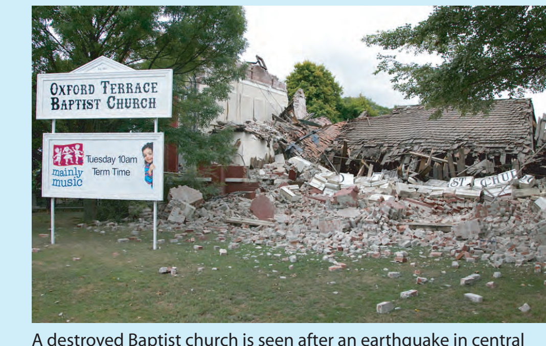
A destroyed Baptist church is seen after an earthquake in central Christchurch February 22, 2011. (REUTERS/Simon Baker/RELIGION)
