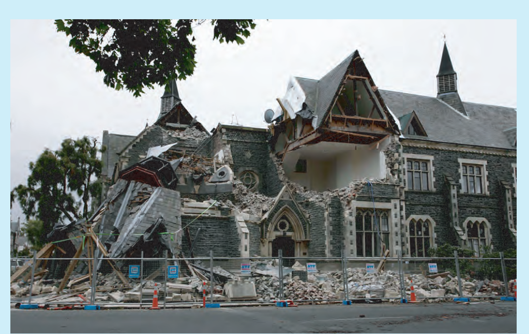
A building in Christchurch, New Zealand, is destroyed after an earthquake struck Tuesday, Feb. 22, 2011. (AP Photo/NZPA, Pam Johnson)
