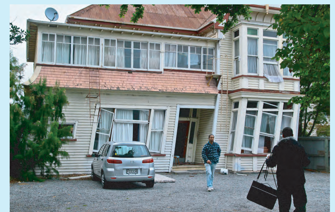
The ground floor of a structure leans perilously, damaged by the earthquake centered near Christchurch, New Zealand on February 22nd, 2011. (© Asher Trafford)
