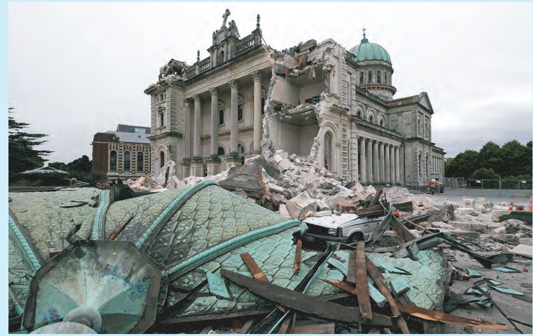
Debris crushed a car outside the Christchurch Catholic Cathedral after an earthquake rocked Christchurch, New Zealand, Tuesday, Feb. 22, 2011. The 6.3-magnitude quake hit at the height of a busy workday, toppling tall buildings and churches, crushing buses and killing dozens of people in one of the country's worst natural disasters. (AP Photo/NZPA, David Wethely)
