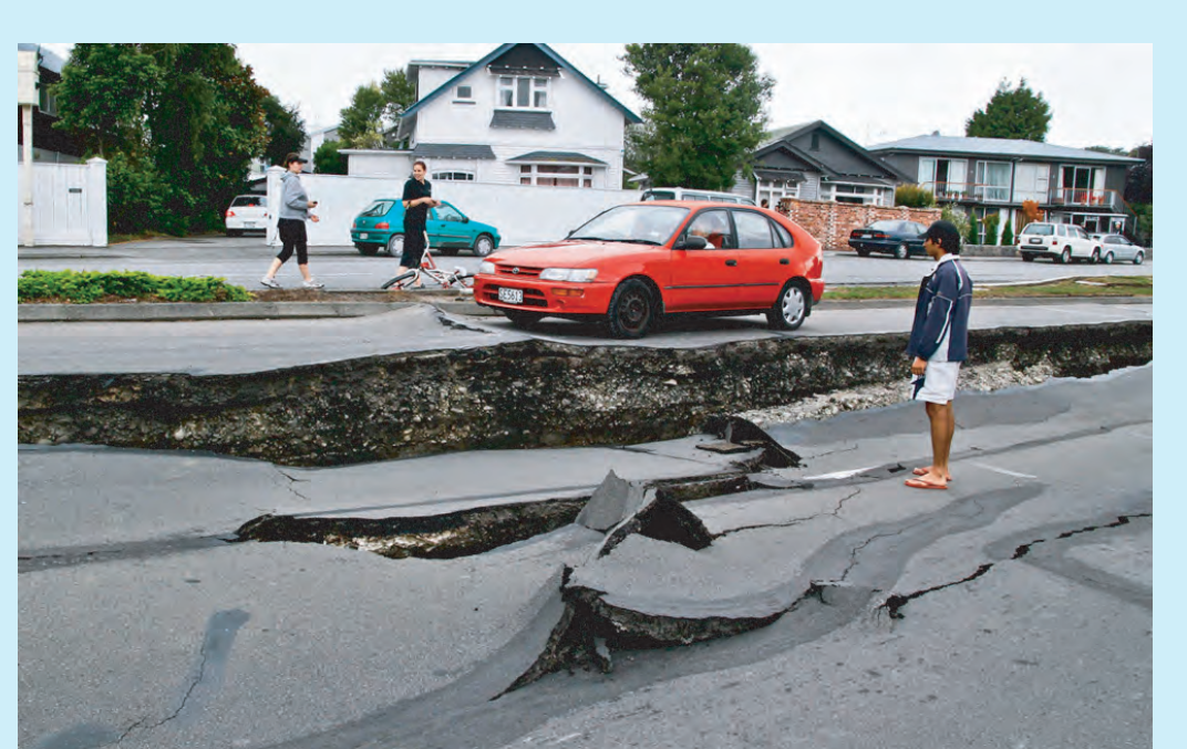
People look at badly fractured pavement after the earthquake in New Zealand on February 22nd, 2011. (© Asher Trafford)
