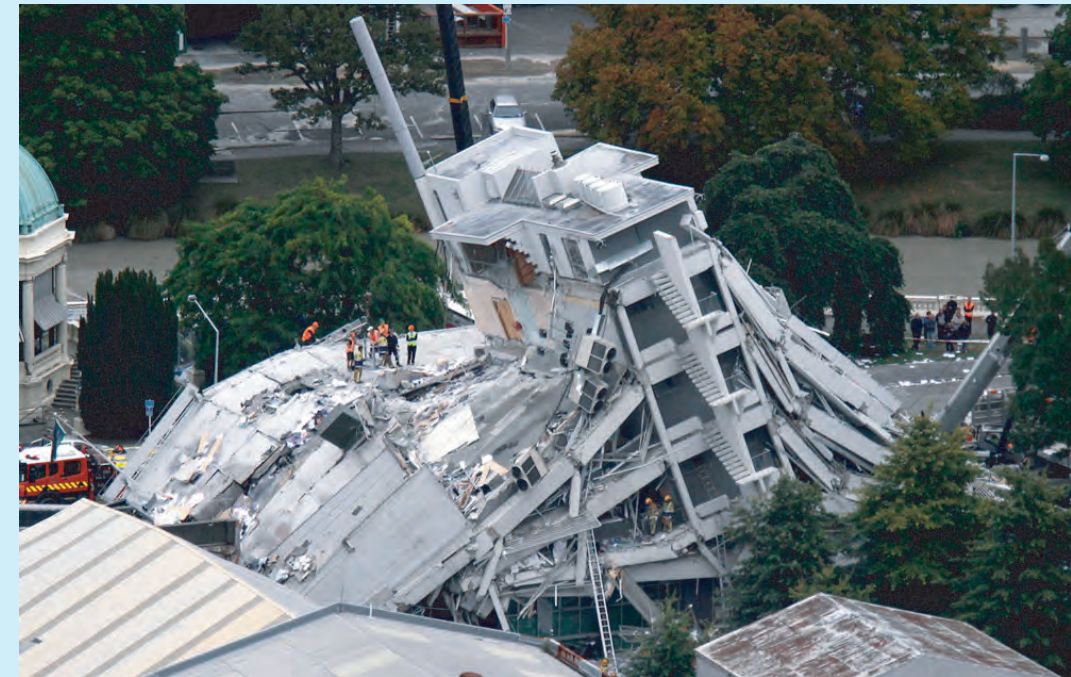
Rescue workers climb onto the collapsed Pyne Gould Guinness Building in central Christchurch, New Zealand, Tuesday, Feb. 22, 2011. A powerful earthquake collapsed buildings at the height of a busy workday, killing at least 65 people and trapping dozens in one of the country's worst natural disasters. (AP Photo/New Zealand Herald, Mark Mitchell)
