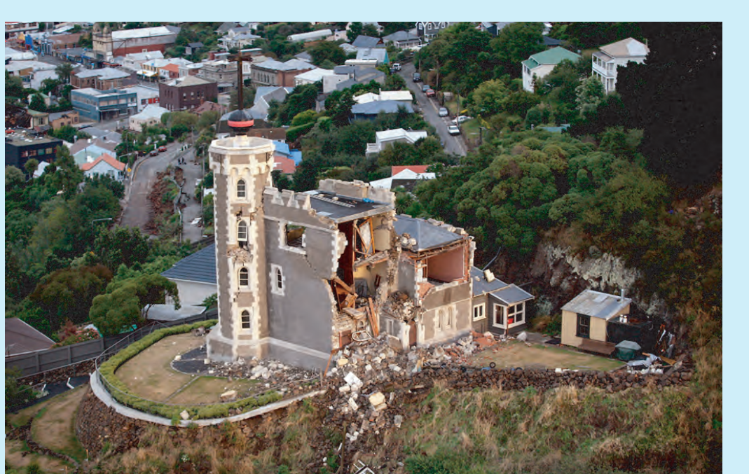
The Timeball Station is seen to be badly damaged, a day after the 6.3-magnitude earthquake in the township of Lyttelton near Christchurch, New Zealand, Wednesday, Feb. 23, 2011. (AP Photo/New Zealand Herald, Sarah Ivey)
