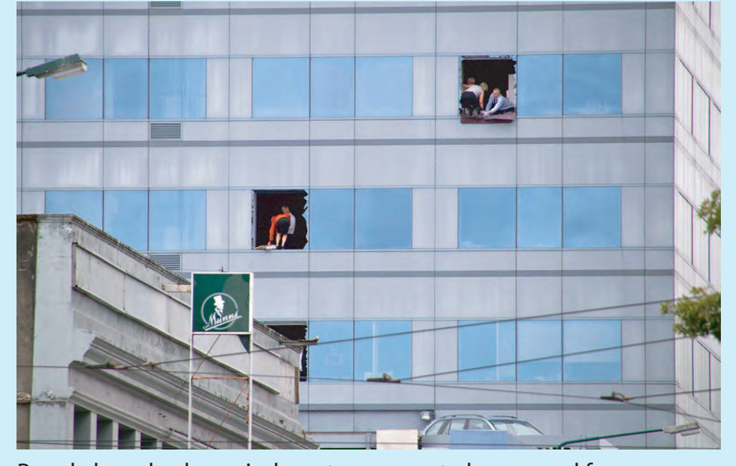
People have broken windows to prepare to be rescued from a high-rise building in central Christchurch, New Zealand, Tuesday, Feb. 22, 2011. (AP Photo/New Zealand Herald)
