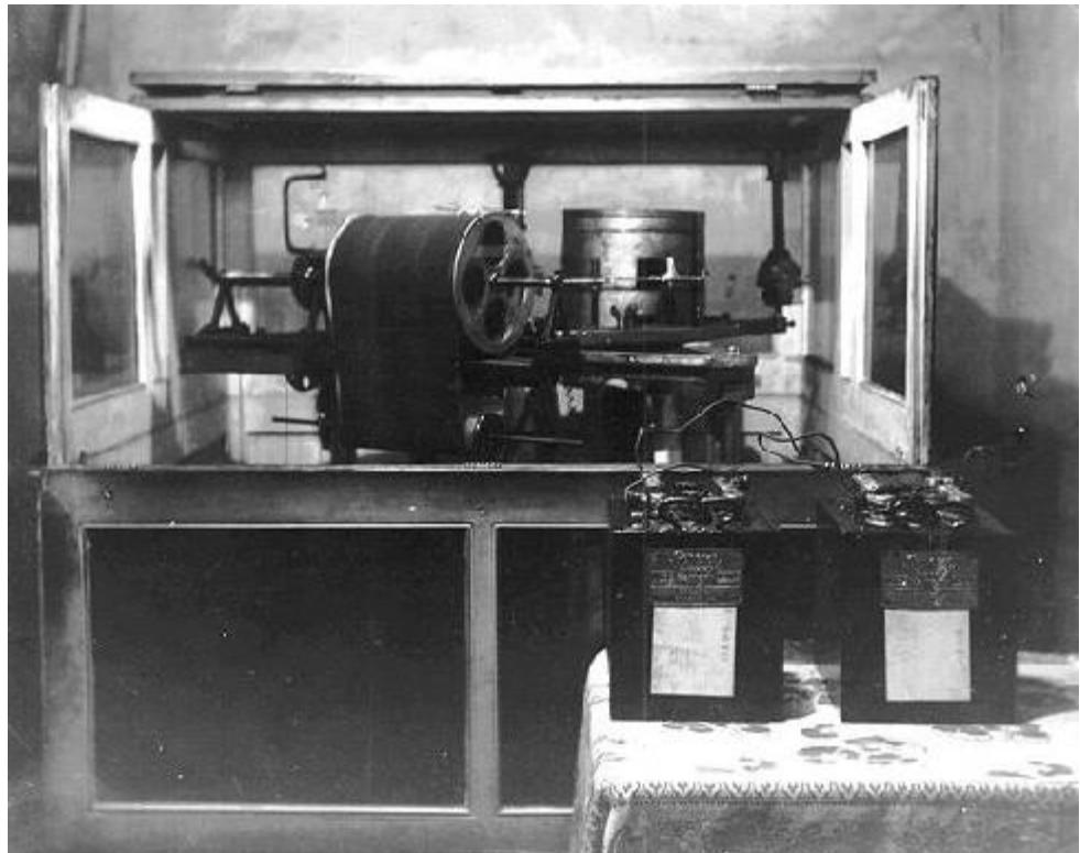
The Wiechert 80 Kg. Horizontal Component Seismograph. Located in the basement of DuBourg Hall at Saint Louis University, the seismograph was installed in 1909 and recorded it's first earthquake on October 9th of that year.
