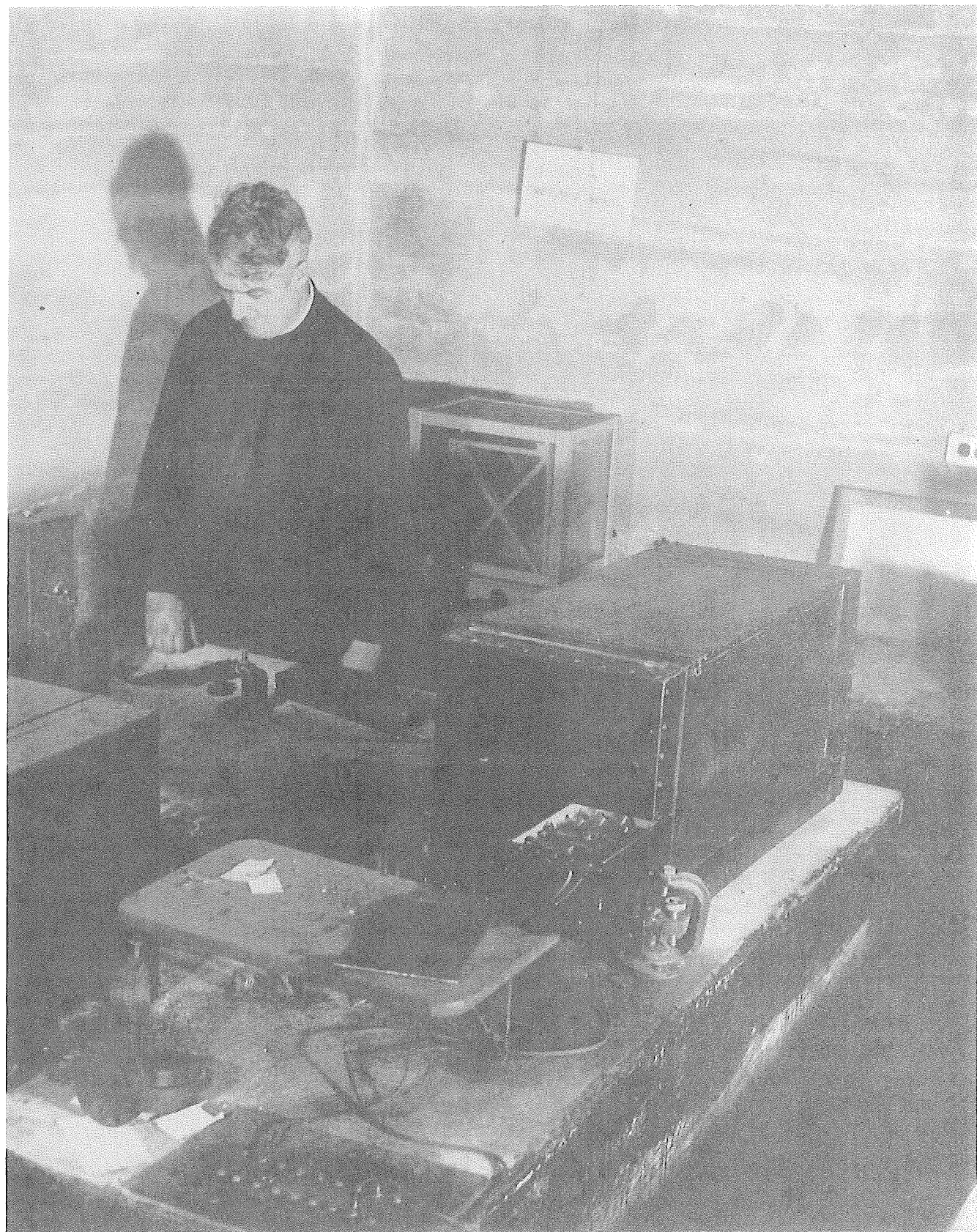
Foreground: Wood-Anderson Seismograph and Recorder Background: Galitzin North-South Component Seismograph Reverend John A. Weber, S. J., Present Director looks on.
