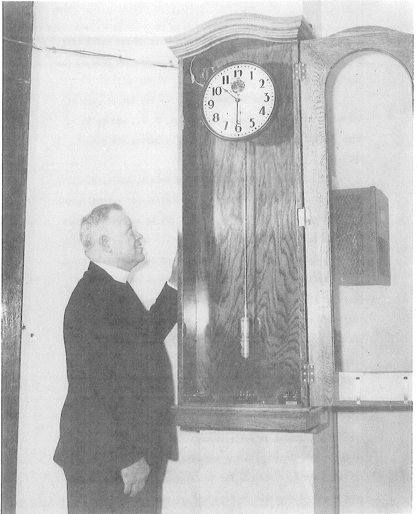
Father Maring Checking the Standard Contact Clock with the Invar Pendulum
