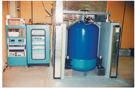
Figure 1 An example of the TT70 type instrument installed at Cantley, Canada, in 1989. The rack on the far left contains the chart recorders and noncritical electronics; the more sensitive components are in the enclosed temperature-controlled rack next to it. The 200 l dewar sits on three feet placed on small granite blocks. The front two feet with the X and Y thermal levelers attached to the dewar bottom are visible. The coldhead is supported from a frame resting on the top of a concrete pier. Normally, the entire SG is enclosed by thermal insulation.
