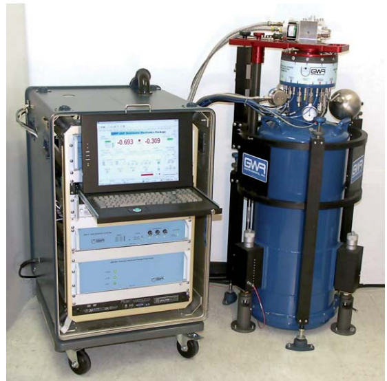
Figure 6 The newest Observatory Model SG and SHI RDK-101 coldhead. All of the control and data acquisition electronics are contained inside one temperature-regulated electronics enclosure. During installation, the front panel is removed and all the controls are accessed by the local keyboard and computer screen normally stored inside the enclosure. After installation, all functions and data retrieval are remotely accessed through an Internet connection. The dewar is 42 cm in diameter and the combined height of the dewar and coldhead is 130 cm.
