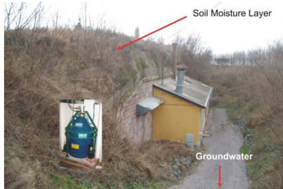
Figure 3. Strasbourg SG, model CO26 in a bunker below the soil moisture level.
